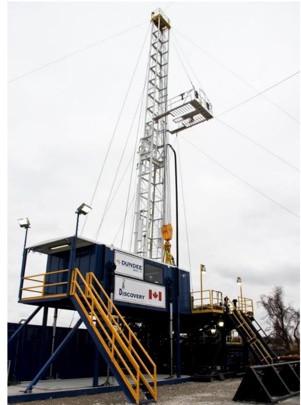
Dundee drilling rig
